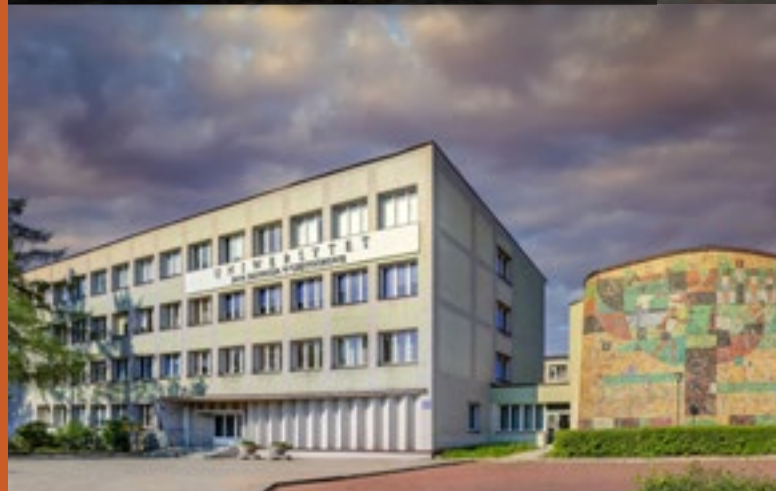
University building at 13/15 Armii Krajowej av.
